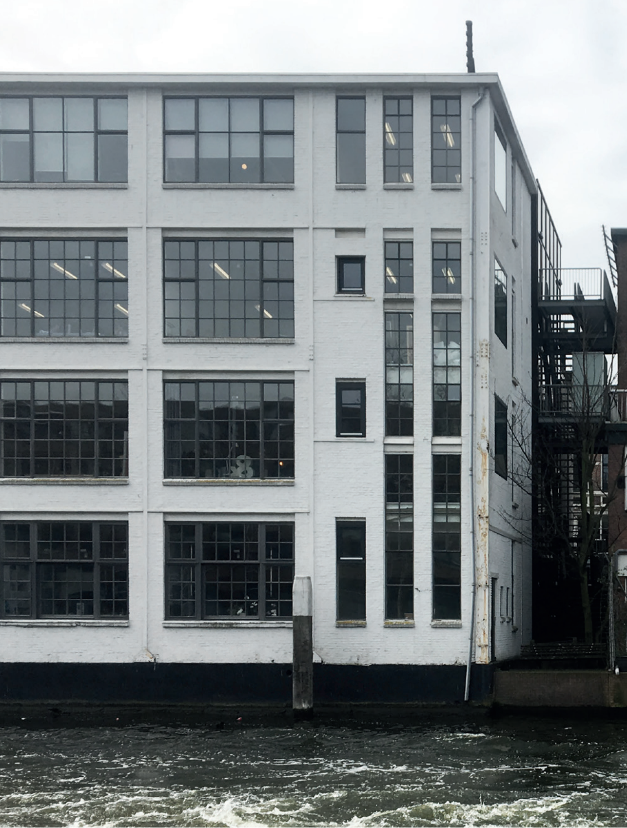
MAKING IS MADE ON MAKING, A TRADITIONAL CANAL ZONE NOW HOUSES SPACE FOR FURNITURE MAKERS / © V SANZ - C.9, N.1, N.4 & N.9
