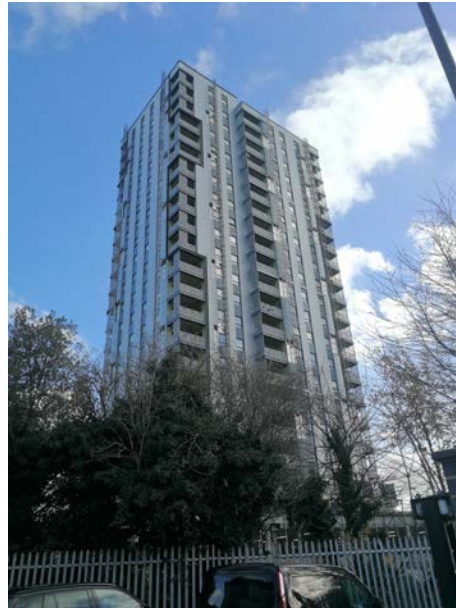
Figure 0.15: A 20-story residential building in NMUH.
