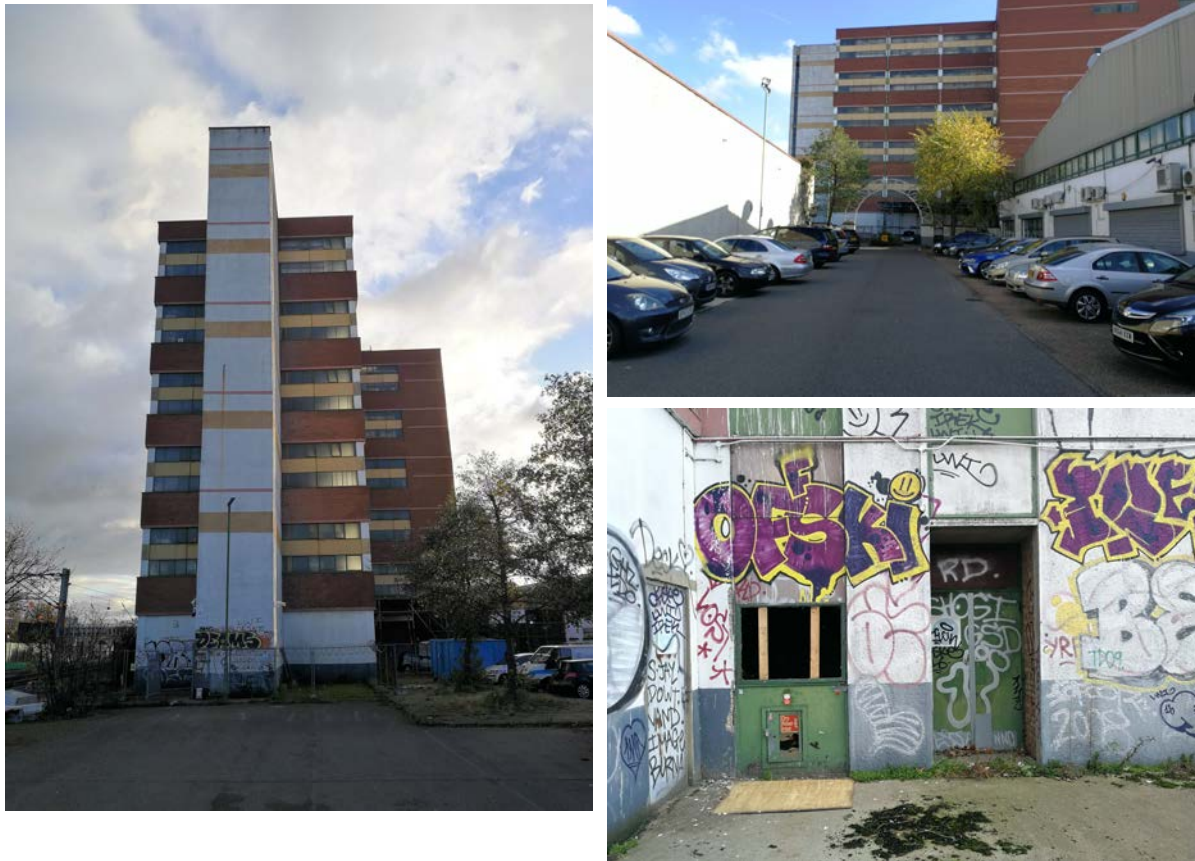
Figure 0.13: Unused or abandoned 1,830-square-metre, 6-story building in MRHCC.
